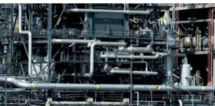
Pipeline and process plant engineering
