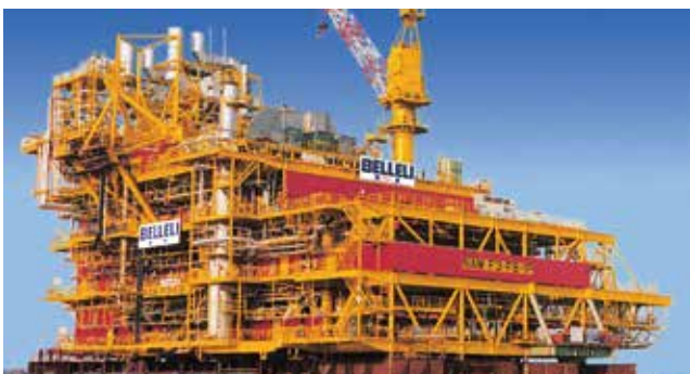
Offshore plant construction: top side
