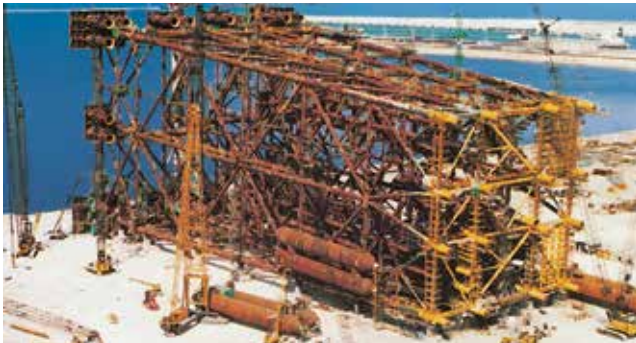
Offshore plant construction: platform
