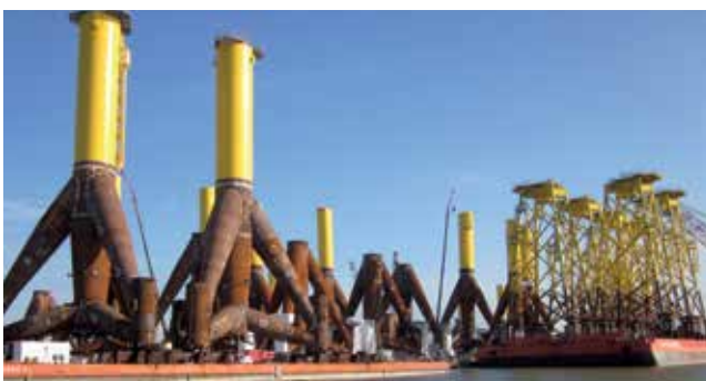
Wind turbine building
